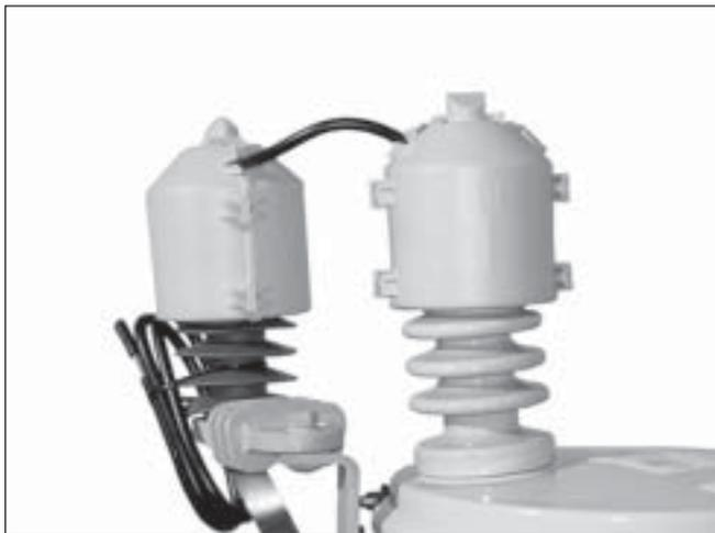
Figure 2: 2163 Wildlife Protectors installed on bushing and lightning arrester of overhead distribution transformer.
